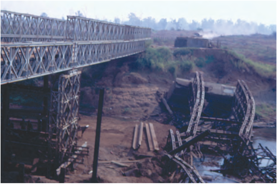
South Vietnamese Army engineers became proficient in repairing and building bridges such as this panel bridge.
